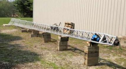
I also cleaned and started putting together the Yagi antenna that goes on the tower. It is a Cushcraft X-7 with the X-740 add on. However, the elements are too long to assemble in the building before mounting it on the tower so that part of the assembly process must wait until the 18' boom is attached to the mast. The task I just completed before writing this was driving in an 8' ground rod next to the pad and connecting it to a tower leg.
